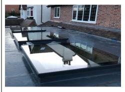
Flat rooflights are available in fixed or electrically openable configurations, and in a range of standard sizes, with either double or triple glazed units.
